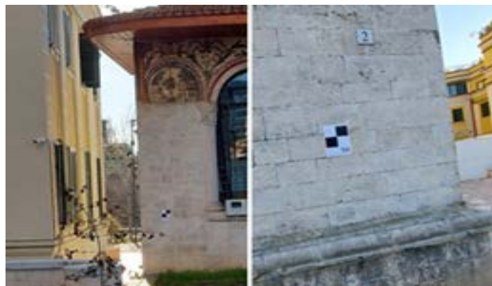
Fig. 2. RAD mark placed on the façade of the object
