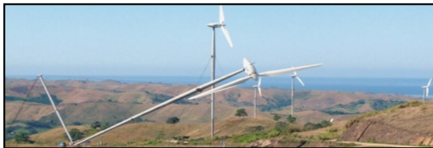
Figure 5: The installation of jack-up wind turbine
