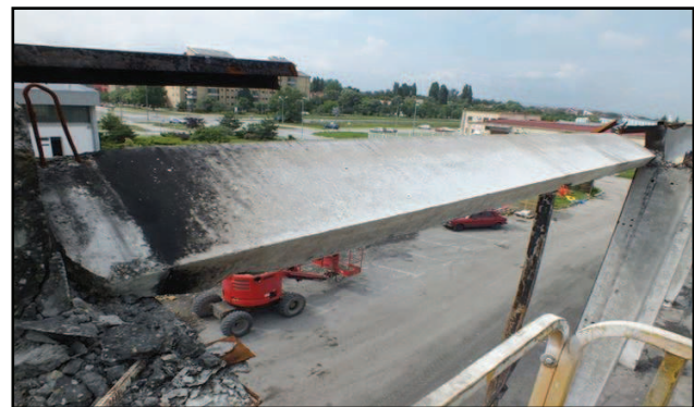
Figure 7: Beam rotation (tends to decline)
