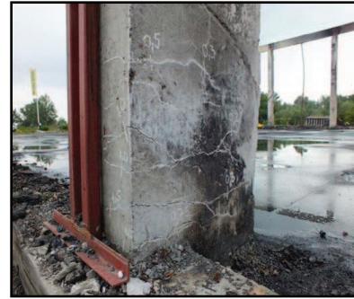
Figure 5: Horizontal cracks due to flexion of column (during the collapse of roof structure)
