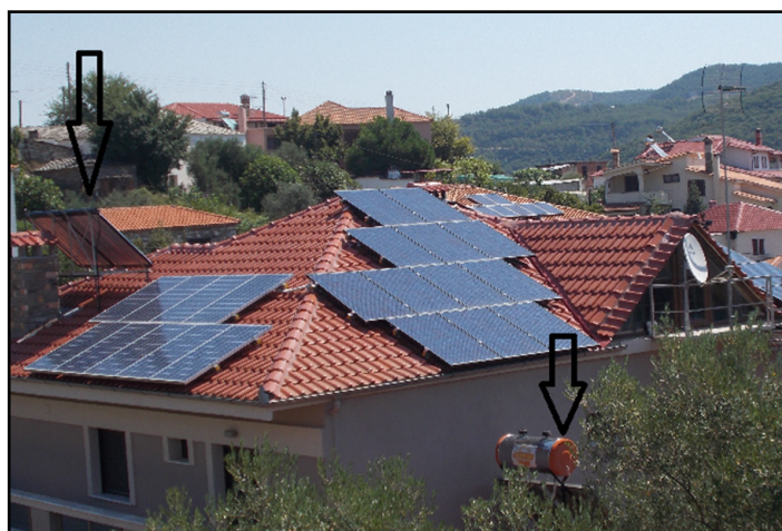
Figure 4: Wrong orientation PV panels
