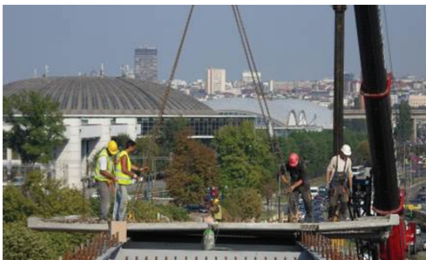
Figure 1: Prefabricated concrete slabs with openings for grouped shear connectors
