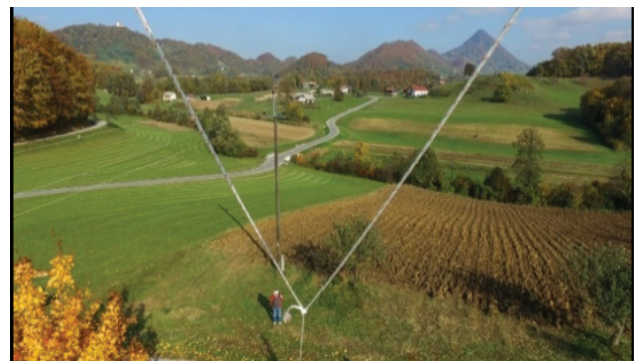
Figure 13. Transporting leader cable for electrical grid
