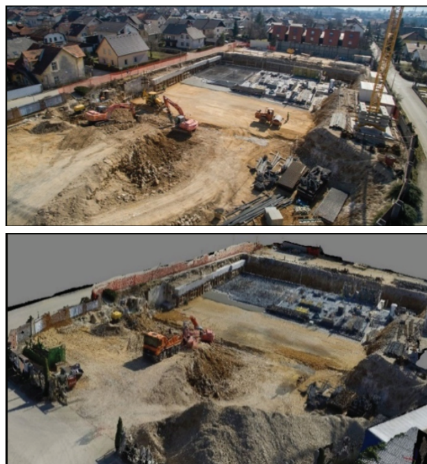
Figure 10: Realistic photography of construction site (upper); 3D model generated from aerial photos using the UAV (lower)
