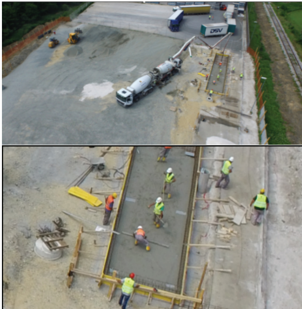
Figure 7: Aerial photograph of the construction site (upper); Magnified picture to monitor the use of protective equipment (lower)
